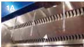
Grease-X-Tractor™ filters, first row of filters
